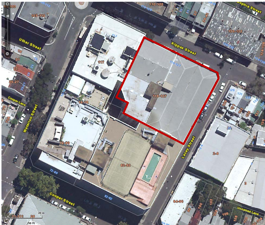
Figure 1: Aerial Photograph showing location of 119-127 Kippax Street, Surry Hills
